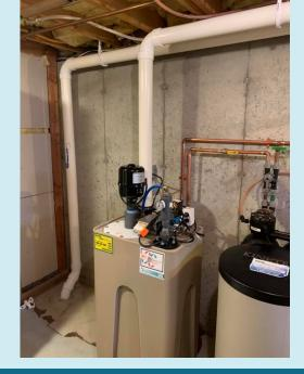
Pictured above is a bubble up system used to remove radon from water. Bubble ups and carbon filters are the two types of systems that can be used to mitigate radon levels in water.
